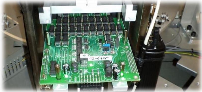
Electrical Function testing
